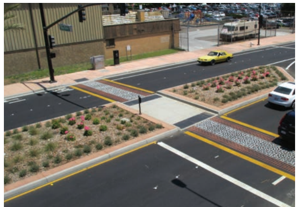
Mid-block crossing near Downtown San Leandro BART Station
