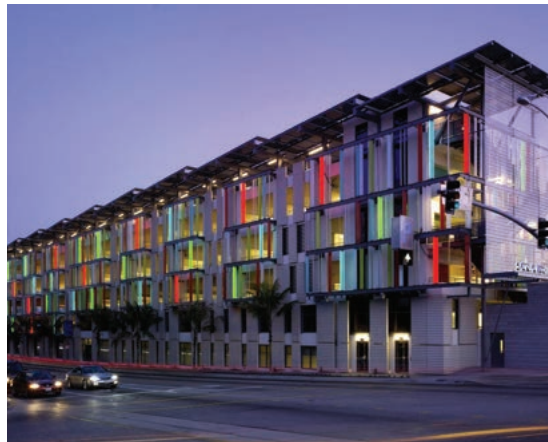
Example of structure parking garage with decorative screening
